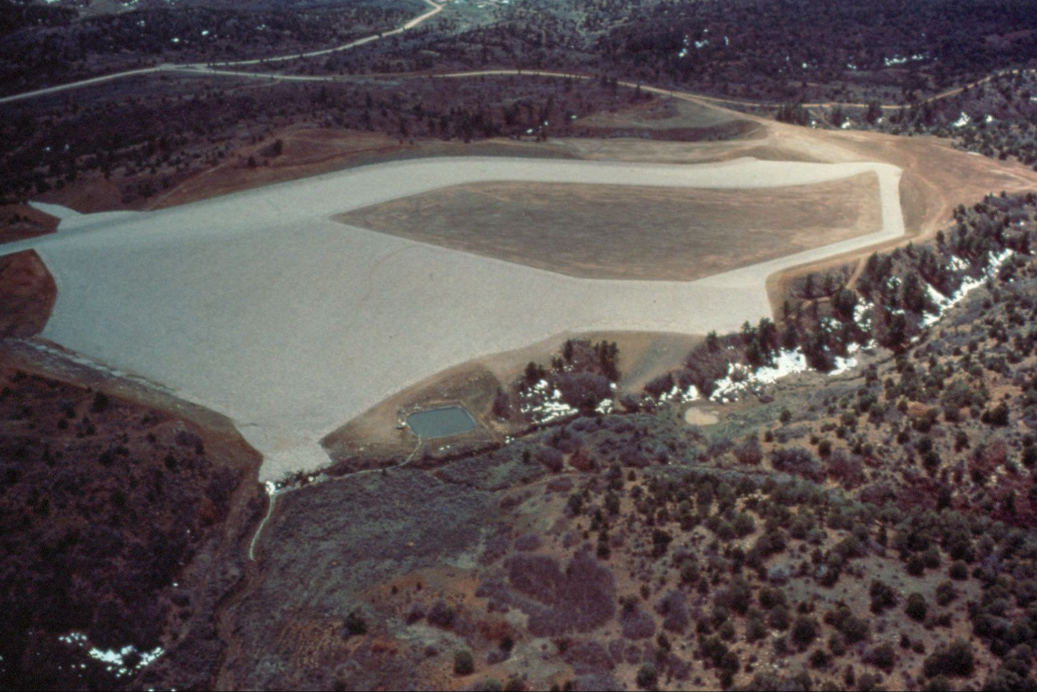
Bodo Canyon alternate disposal site, 12 km from Durango, Colorado, USA, 1992
